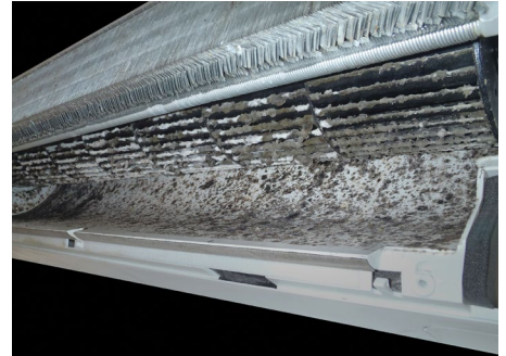
Mold thrives on mini-split blower wheels
